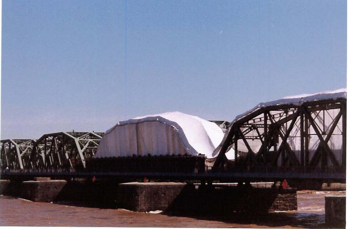
Cable Supported/Metal Deck Platform System & Containment
