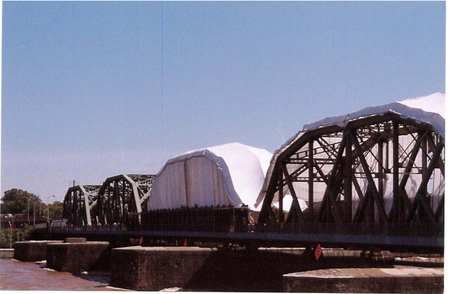
Cable Supported/Metal Deck Platform System & Containment
