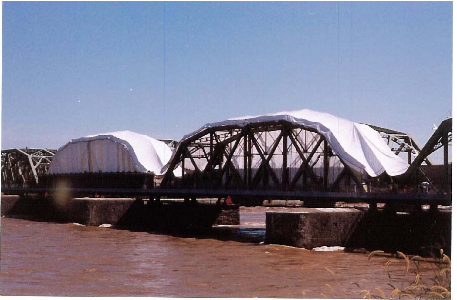
Cable Supported/Metal Deck Platform System & Containment
