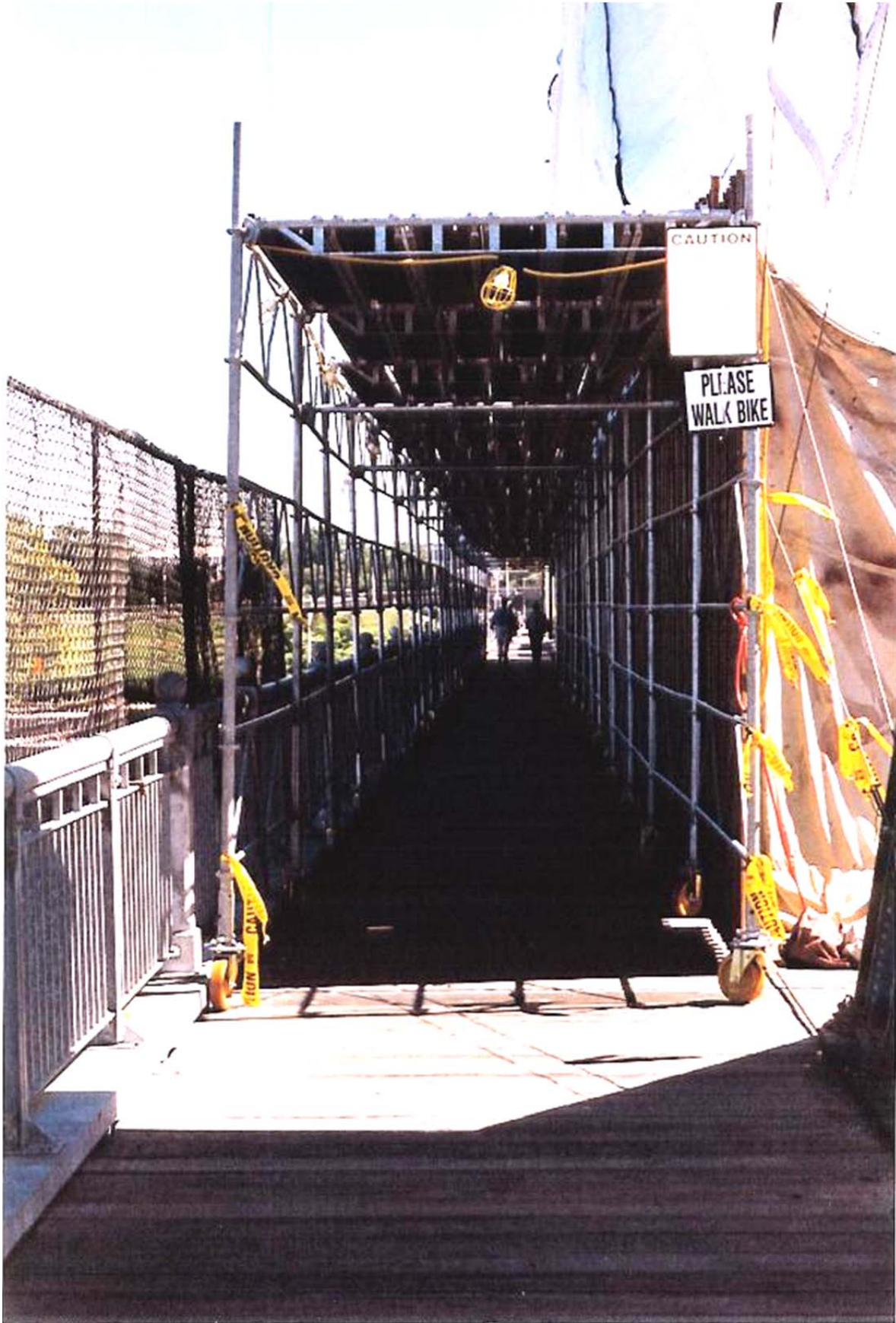
Scaffold Walkway System
